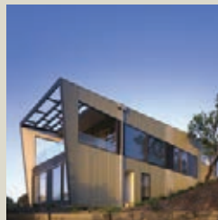
Roof and walls: COLORBOND® steel in a range of colours
