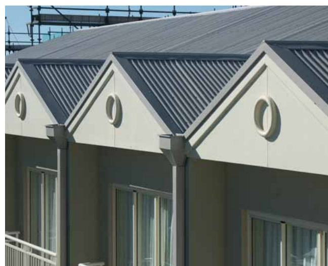
Figure 3.6.1 Typical transverse flashings
